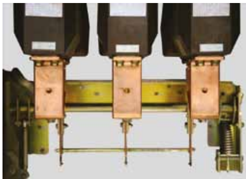
Drawing 15. Earthing switch open
