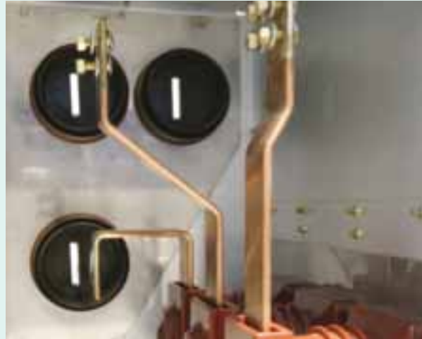
The structure of busbar compartment with rated current 1250A and rated short-circuit breaking current 25kA
