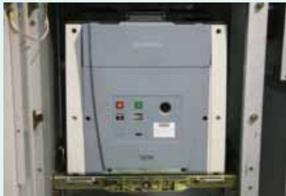
Suitable for rated short-circuit breaking current \geq 31.5\text{kA} and rated current \geq 3150\text{A} with classic breaker
