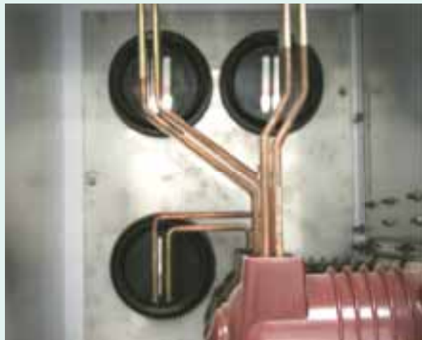
The structure of busbar compartment with rated current 2500A and rated short-circuit breaking current 25/31.5kA
