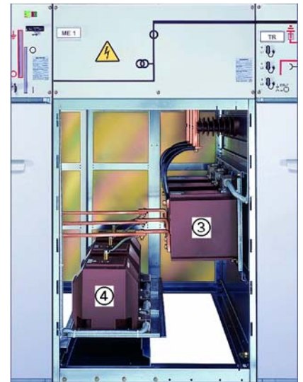
Fig. 25: Block-type current transformers and voltage transformers in the billing metering panel
