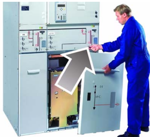
Fig. 30: Interlocking of cable compartment cover (cable compartment cover removed in earthed circuit-breaker panel)
