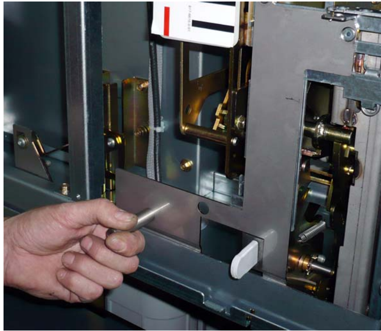
Fig. 91: Fitting the locking device
