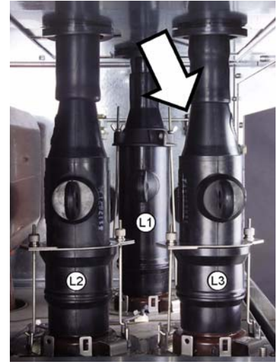
Fig. 24: Cable routing to the top
