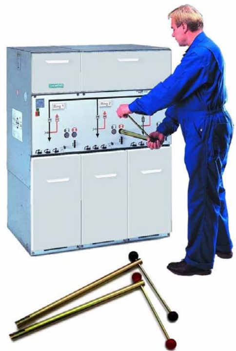
Fig. 30: Rotary lever with red handle for earthing and de-earthing, with black handle for load breaking
