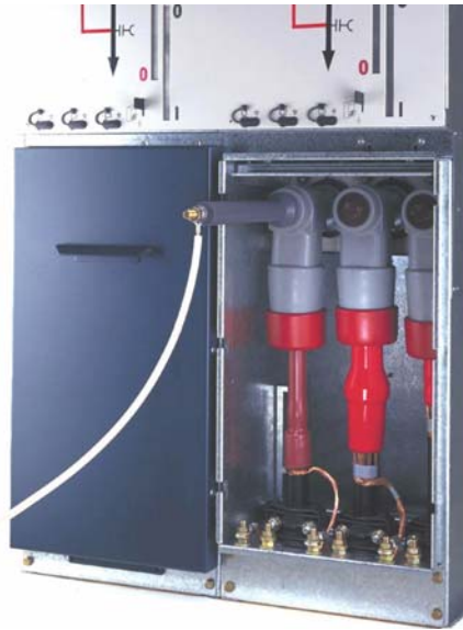
Fig. 32: Mounted test adapter
