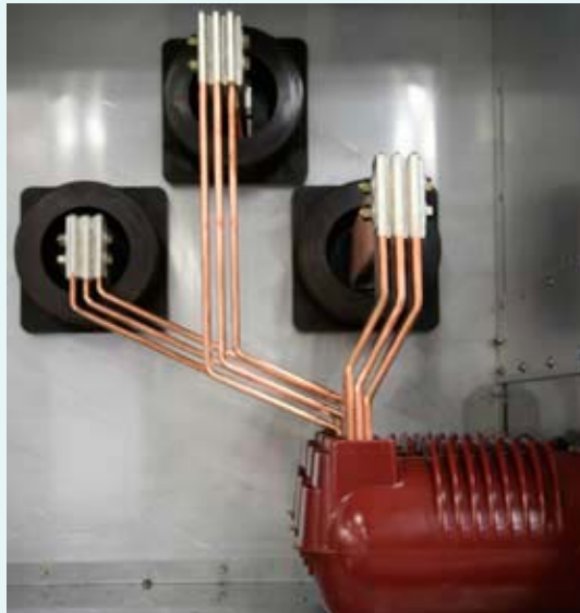
Busbar compartment with rated current 3150A
